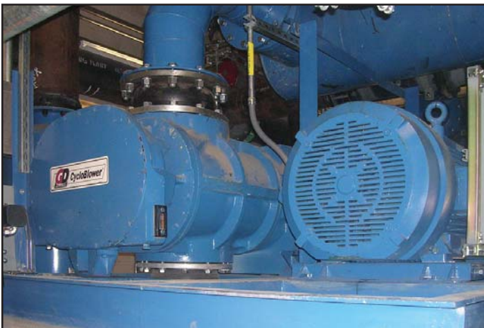
250 HP Cycloblower Package with special ductile iron drive
